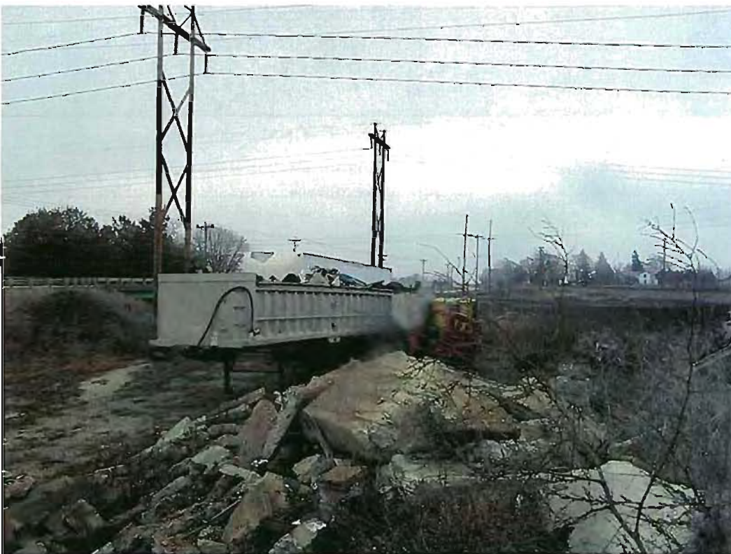
Date:02-10-2012 Time: 11:28AM Direction: Northeast Photo by: Jen O'Hearn Exposure #: 022 Comments: View of open top trailer with waste visible inside.
